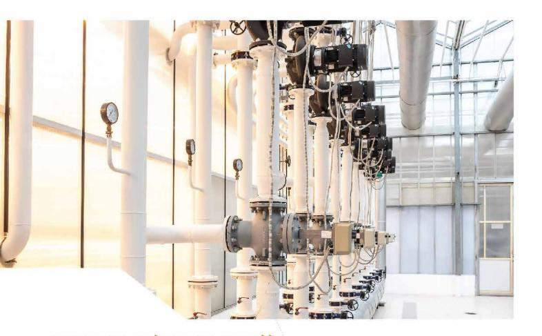
The heating system design is based on the climatic conditions of the greenhouse complex location according to SP and SNIP. Compensation of heat losses is provided by the circuits of heating systems with separate regulation of each circuit. The heat carrier quantity for each heating circuit is calculated automatically, taking into account the temperature and time limits set pursuant to requirements of the plant growing technology.
