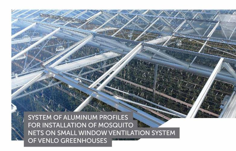
The system is fully adapted to a standard roof, which became possible due to the development of new profiles and small windows. This enables easy installation of cassette-type mosquito nets with different cell size.
