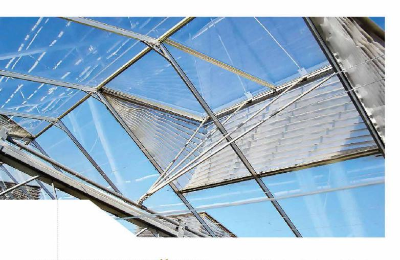
The holder has a box shape, which, when the small window is closed, allows the mosquito net to be protected from precipitation and atmospheric influences. For normal operation of the small windows and adaptation to the existing roof, a new ridgy frame bar was developed.
