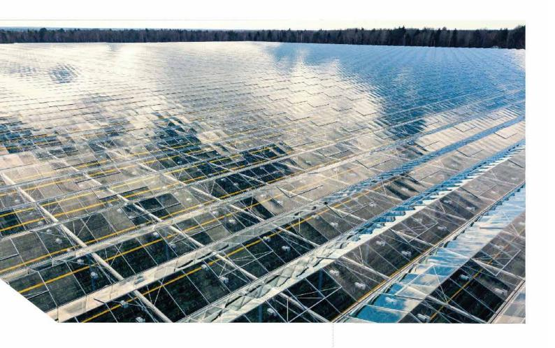
The small window ventilation system of industrial greenhouses is designed for natural exchange of the greenhouse enclosed air volume and the outside air through the vents in the roof of the transparent enclosure for the 4th generation complexes.
